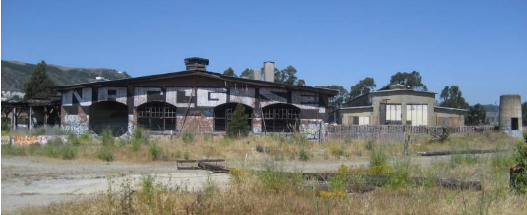
Extant Historic Railroad Buildings. Looking northwest (facing away from the Caltrain tracks), the Roundhouse is on the left and the Lazzari Fuel Company building is on the right.
