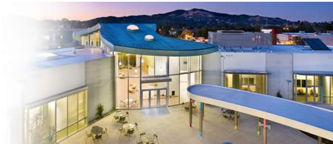
Figure 61. The innovative Marin Health and Wellness Campus brings a spectrum of services and clinics together in one inviting place. It is a result of local individuals, organizations, businesses, and government pulling together in the spirit of cooperation and neighborhood revitalization. The project involved the design and renovation of approximately 74,000 square feet in five buildings. https://www.marinhhs.org/marin-health-wellness-campus
