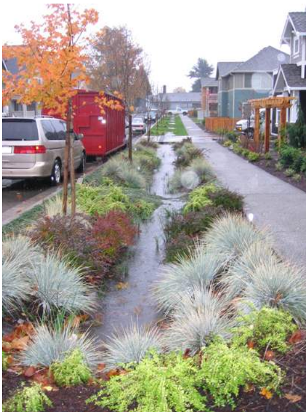
Figure 44. Green infrastructure such as bioswales are example to treat stormwater runoff. http://water.epa.gov/infrastructure/greeninfrastructure/gi_what.cfm
