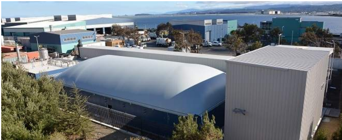
Figure 17. In partnership with Blue Line Transfer, Inc. – Sunset Scavenger has designed and developed the Blue Line Biogenic CNG (compressed natural gas) facility to produce over 100,000 diesel equivalent gallons of CNG per year. http://zerowasteenergy.com/what-we-do/our-projects
