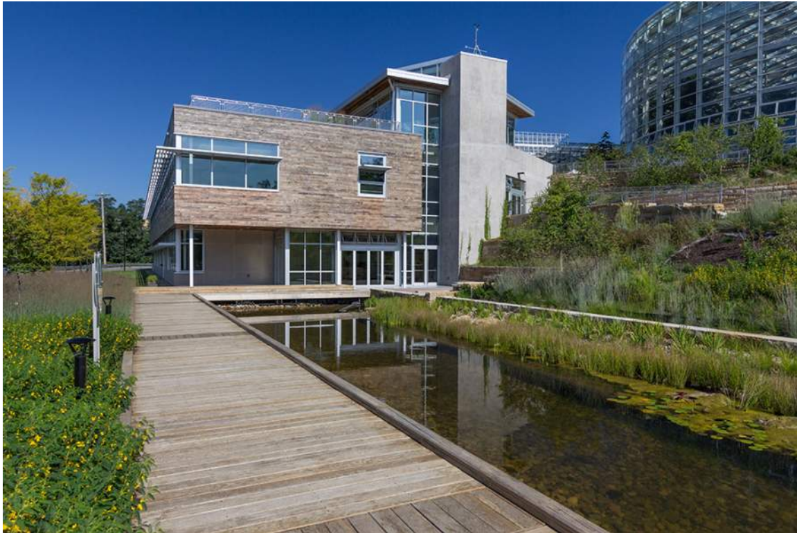
Figure 40. Phipps Conservatory and Botanical Gardens (Pittsburgh, Pennsylvania) has a goal of enhancing wetlands and reducing water use in the buildings. http://www.world-architects.com/en/projects/42835-Phipps-Conservatory-and-Botanical-Gardens-Center-for-Sustainable-Landscapes
