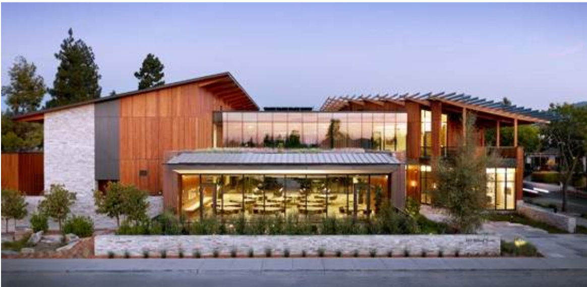
Figure 12. The David & Lucile Packard Foundation Project in Los Altos, California achieved Zero Net Energy certification in 2013. http://www.packard.org/about-the-foundation/our-green-headquarters/
