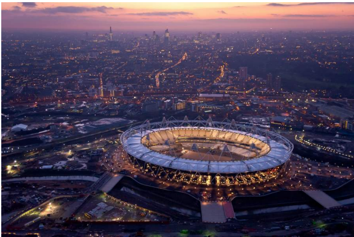
Figure 4. The London 2012 Olympic and Paralympic games is a great example of a sustainable approach, using the One Planet Living framework by Bioregional. Remediating a contaminated brownfield site, the City of London & Bioregional said "we want to build on that contribution by helping organizers of sports events to reduce environmental impacts, boost the local economy and help surrounding communities to secure long term benefits." http://www.bioregional.com/one-planet-sport-3/
