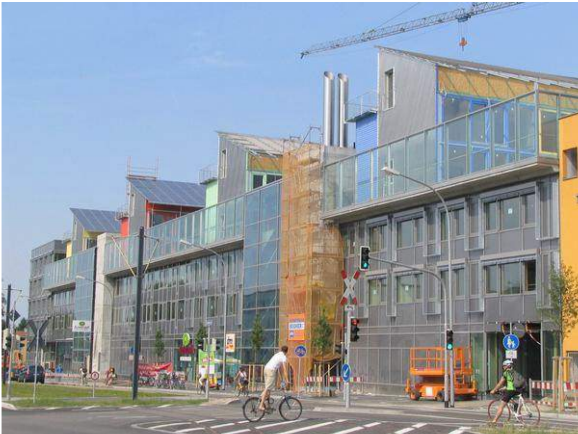
Figure 7. Four and five-story buildings can now produce more energy than they use, Freiburg, Germany http://www.theguardian.com/environment/2008/mar/23/freiburg.germany.greenest.city
