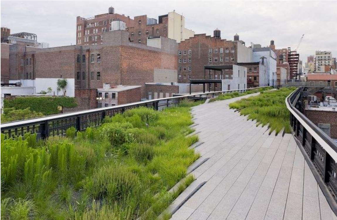
Figure 53. The Hudson Yards project located at New York City's railyard and its neighbor, the Highline Park project, are both milestones in sustainable building, adaptive reuse. Hudson Yards also features a pneumatic vacuum waste elimination tube system.
