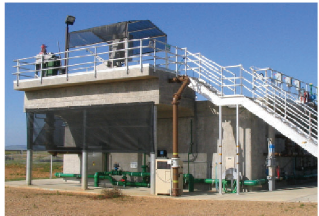
The image above shows a water recycling facility similar to the one included in the Baylands design. (Image Source: Brown and Caldwell)
