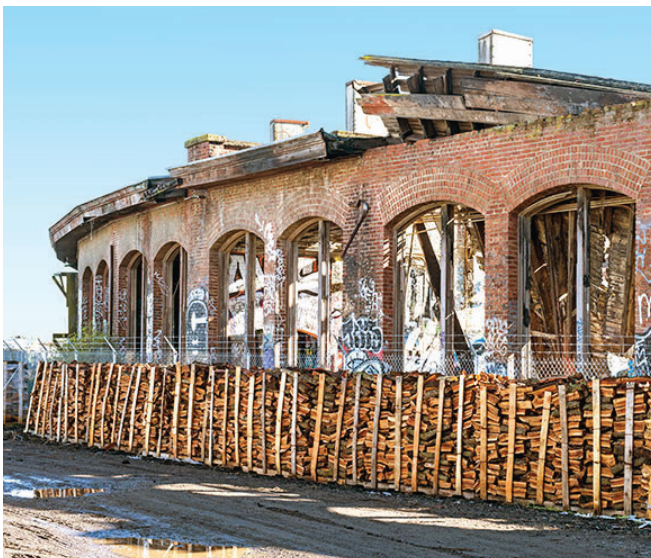
The current condition of the historic Roundhouse building.
