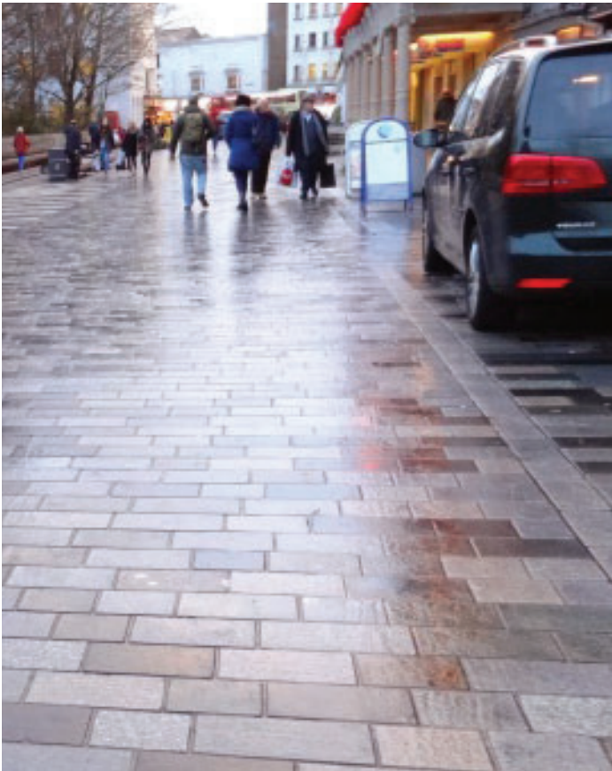
Continuous Signature Paving into Roadway
