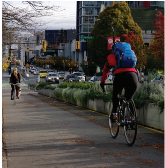
Example of a Class IV protected bike lane which provides connections for all ages and abilities and encourages travel by bicycles and micro-mobility devices.
