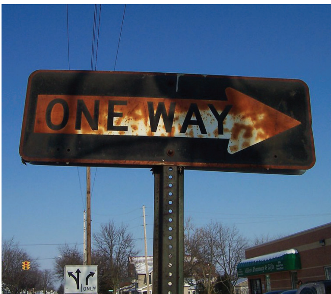
Signs that are not properly maintained
