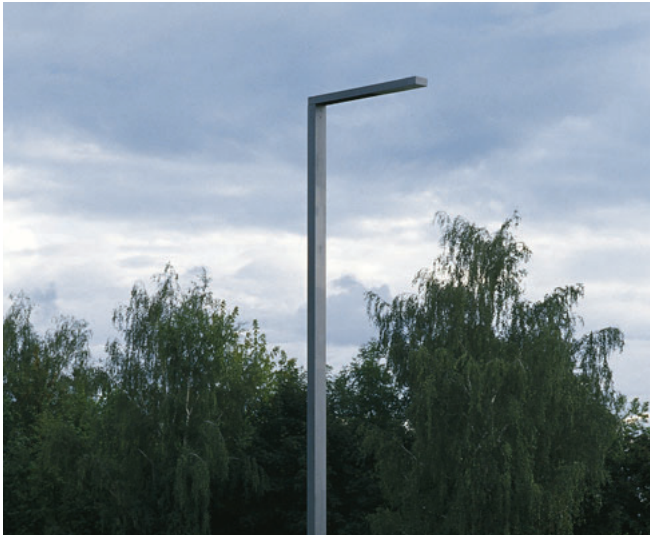
Road Light Pole
