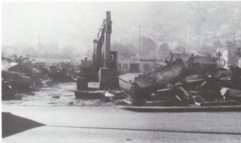
The wrecking crew razed all the buildings in one morning
