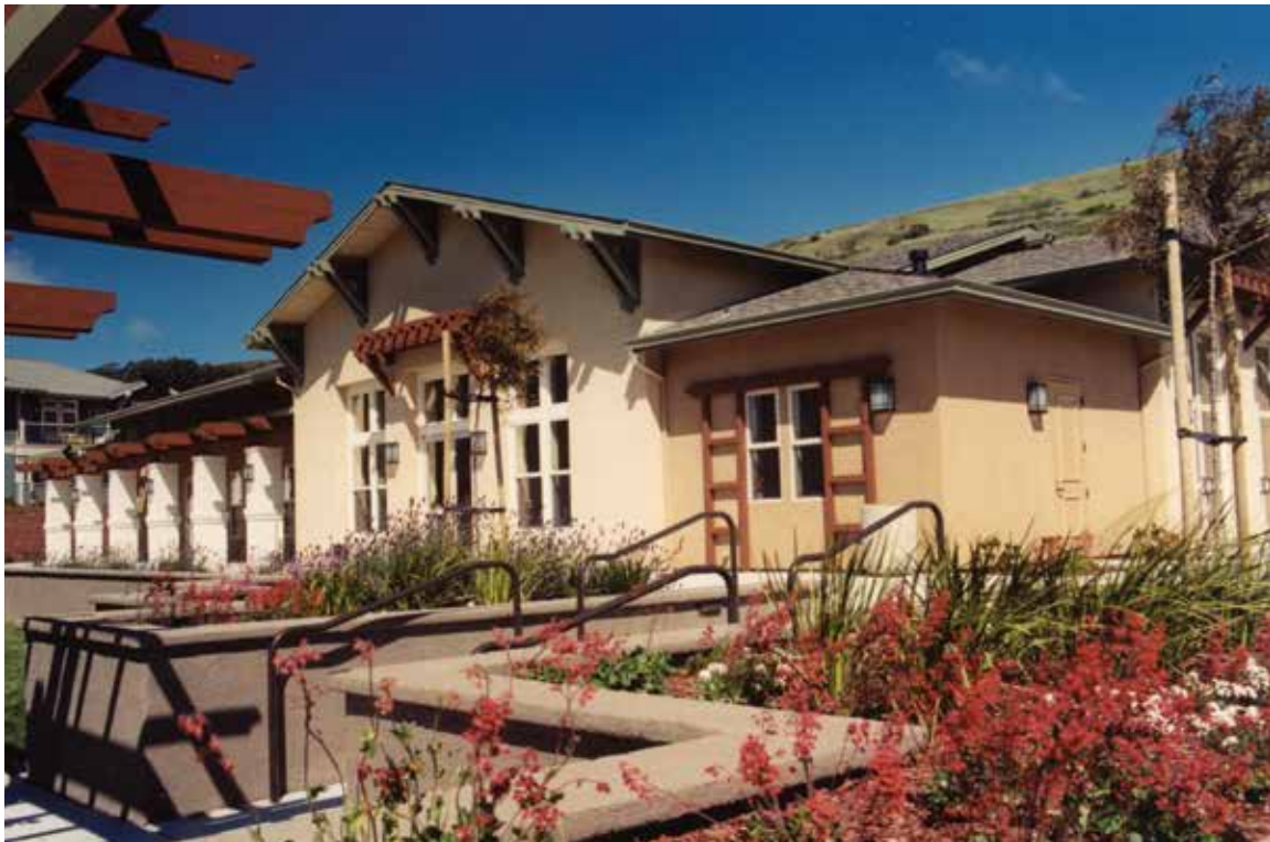
Built with funds provided by Northeast Ridge developer Brookfield Homes and designed with professional arts venues in mind, the Mission Blue Center quickly became a focal point for Brisbane's artists and performers. The facility's unique acoustics and beautiful setting have become known far beyond Brisbane's borders.
