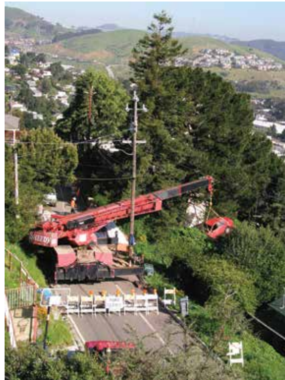
Six weeks of rain in the spring of 2006 saturated the hillsides supporting many Brisbane homes, turning earth into mud. On April 11, a mudslide on Humboldt Road carried off one unoccupied car and damaged three homes. On April 20 a crane removed the car.
