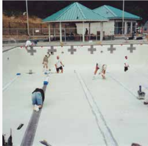
The pool, under construction in 2000.
