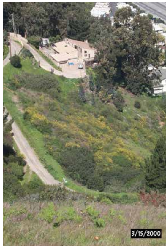
This lot in Brisbane Acres demonstrates both the desirability of preserving the mountain habitat and the severe challenges of trying to build on the property.
