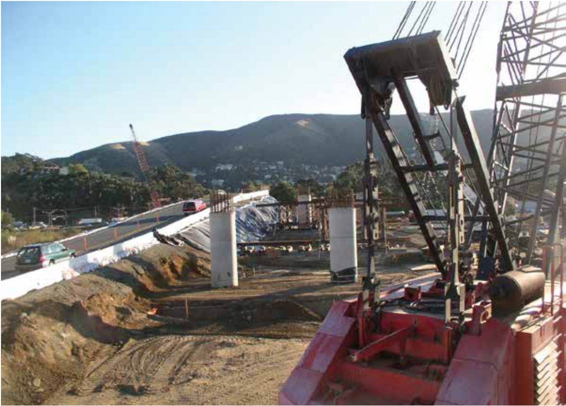
New Tunnel Avenue Bridge under construction, 2007.
