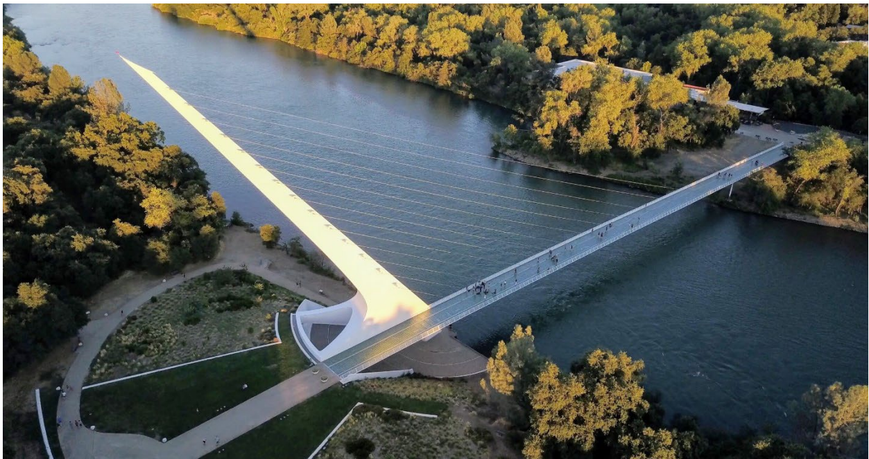
Sundial Bridge by Santiago Caltravas, Redding, California
