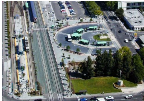
Off-street shuttle stop and passenger loading, transit, bike parking, shelter, retail, shared platform for Caltrain and light rail
