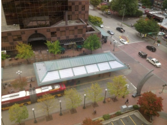
Converted street into bus facility, public plaza
