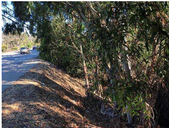
Shoulder of northbound Bayshore Boulevard approximately 225 feet north of Valley Drive.
