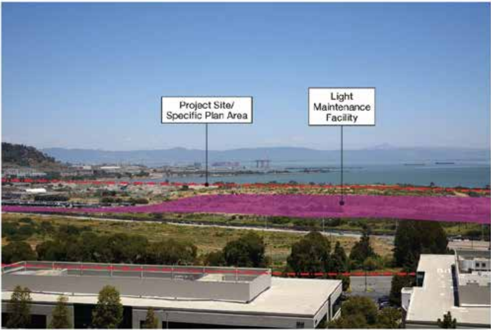
Viewpoint H: Mission Blue Drive off Guadalupe Canyon Parkway (Northeast Ridge), facing east
