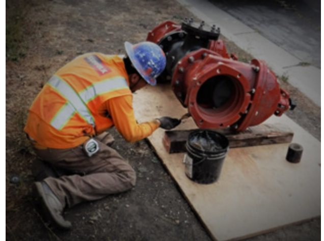
Water Main Replacement Project on Kings last year.
