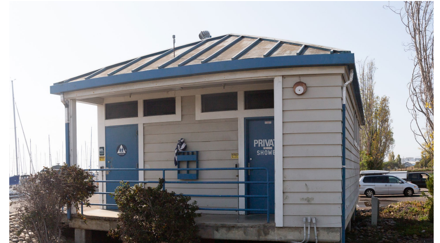
Marina bathrooms. Critical infrastructure for those living on boats at the marina. Private to marina users.
