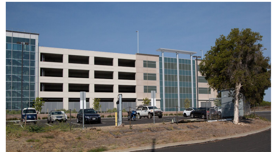
EV charging station in parking lot near Harbormaster's Office.
