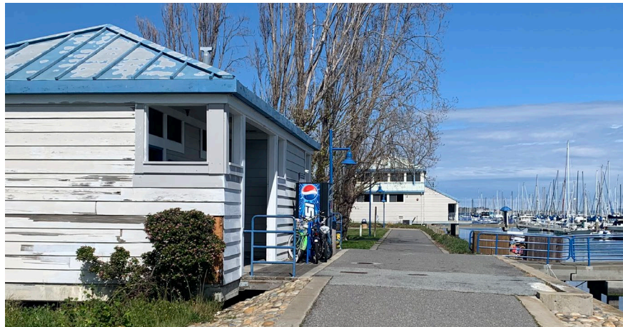
Marina restrooms, trash cans at head of gangway with the Harbormaster's Building beyond.
