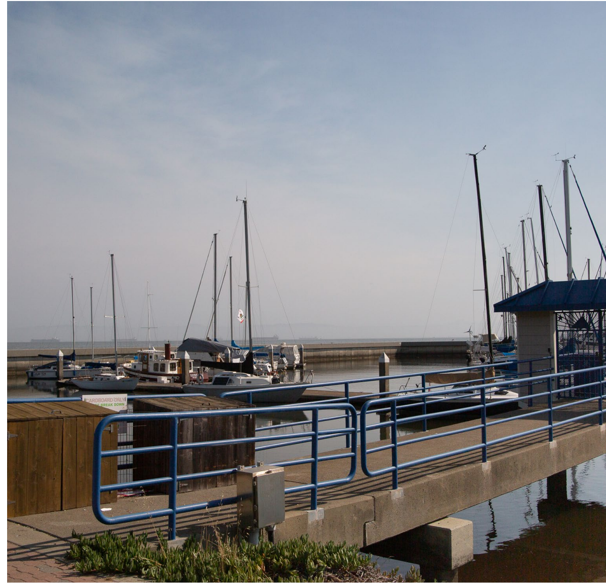
Gangway to Dock 6 with concrete breakwater beyond.
