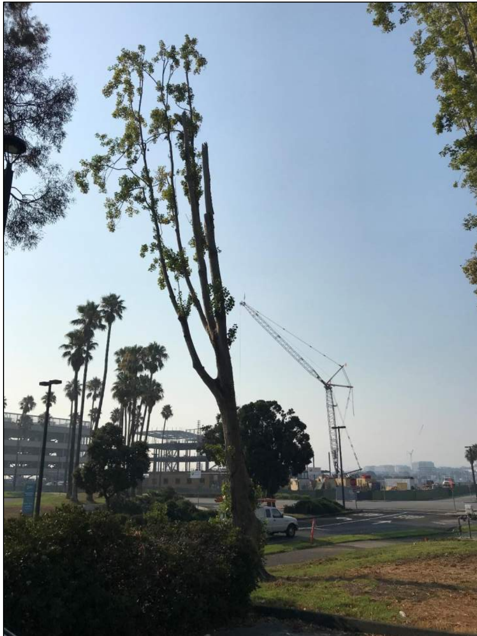
Tree #20: 63.8-inch circumference poplar with significant decay in trunk and roots
