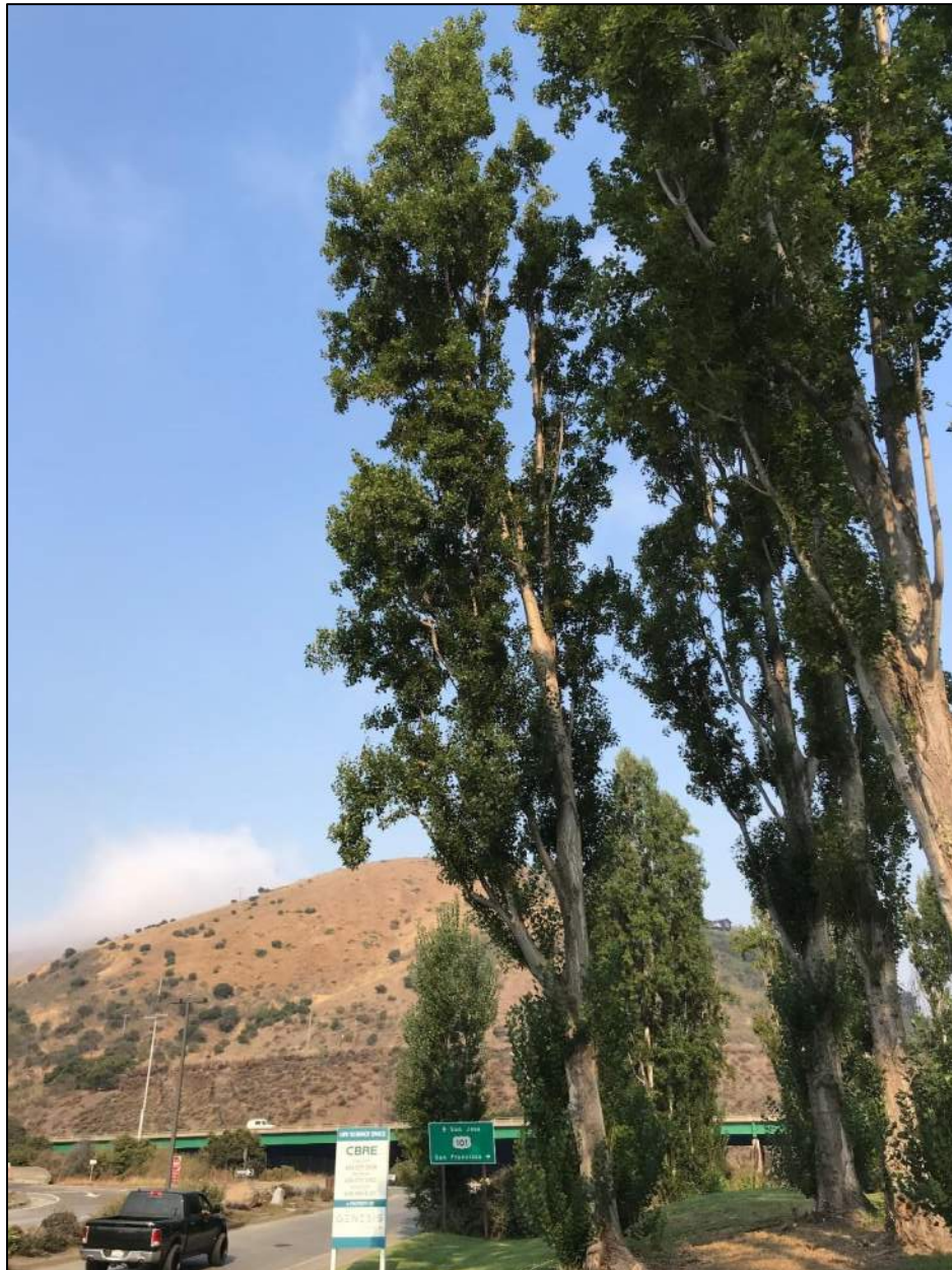
Tree #14: 85.5-inch circumference poplar with significant decay in trunk and roots
