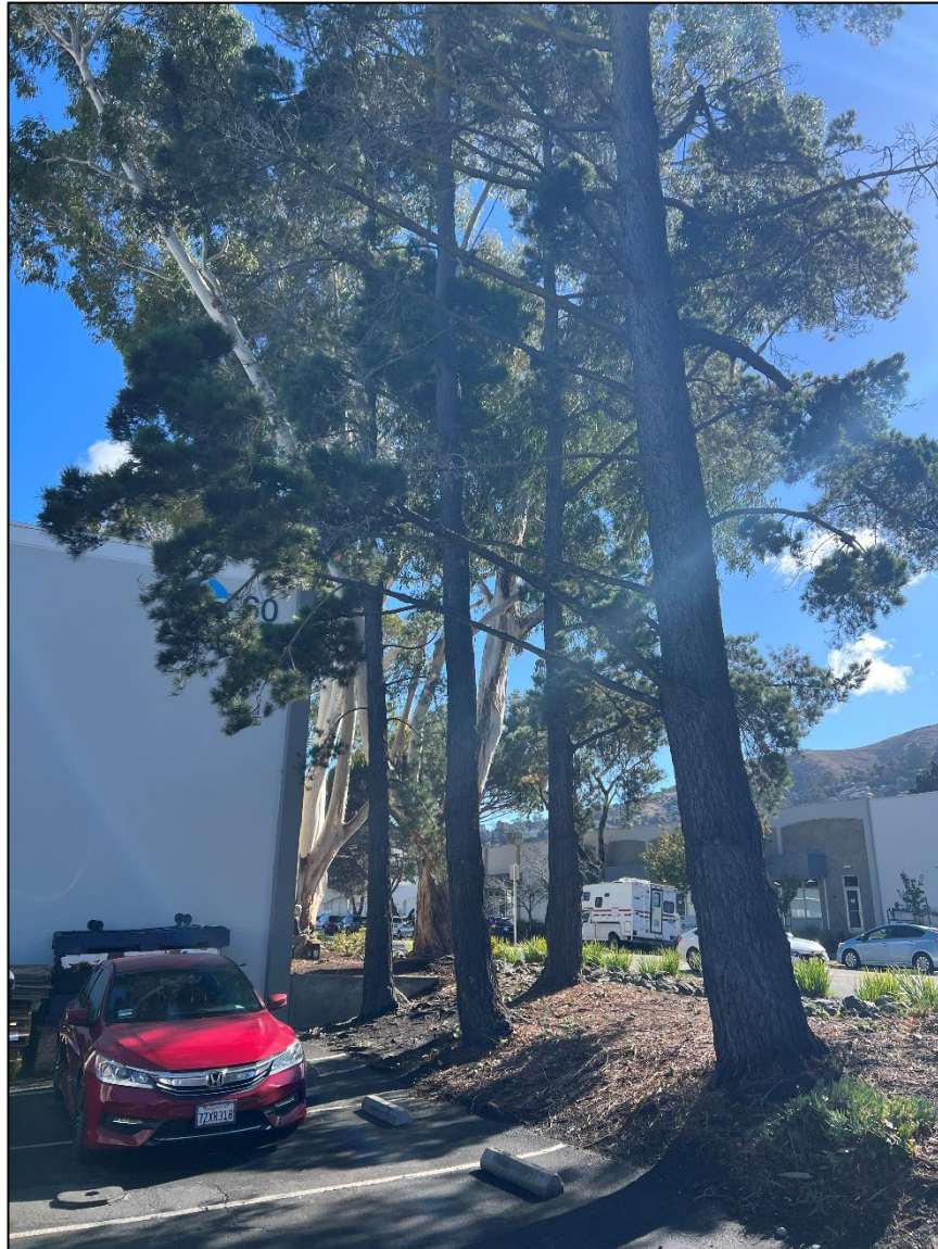
Photo 3: Subject Monterey pine (center) growing amongst a cluster of other pine. Its canopy was overhanging the parking lot.
