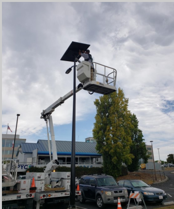
New light poles being installed.
