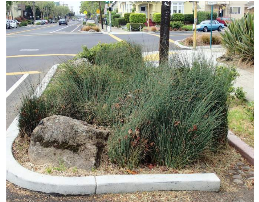
Bulbouts at key intersections should be built where feasible to reduce pedestrian crossing distances.
