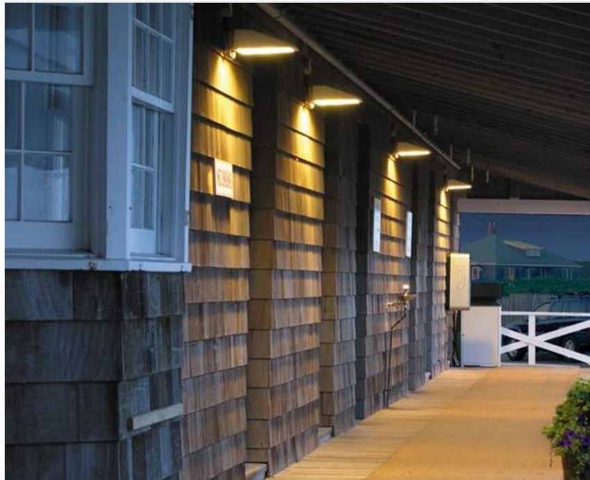
Commercial lighting should be Dark Sky compliant.
