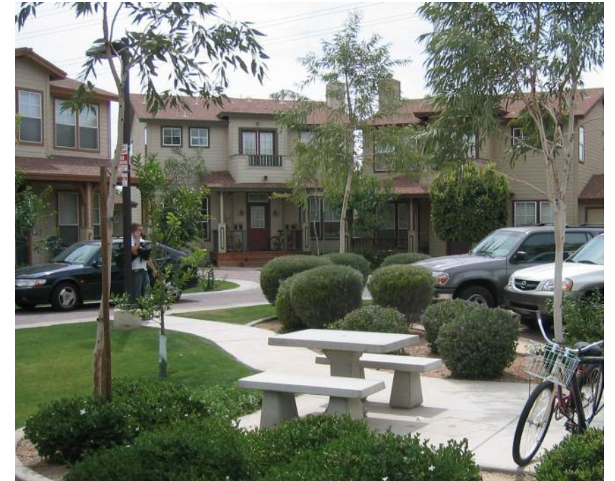
Garages and parking areas shall be oriented toward the center of development sites.
