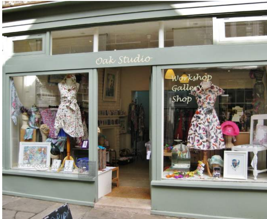
The glazing along primary shop fronts should occupy at least 75% of the first floor wall area, and should provide clear views of merchandise
