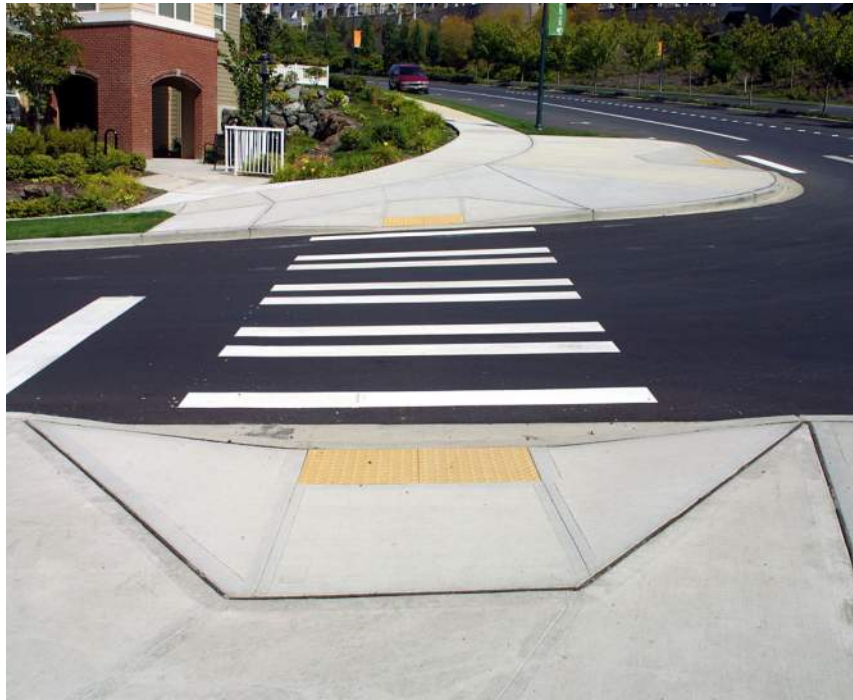
Curb ramps should be parallel to the direct path of travel across the intersection.
