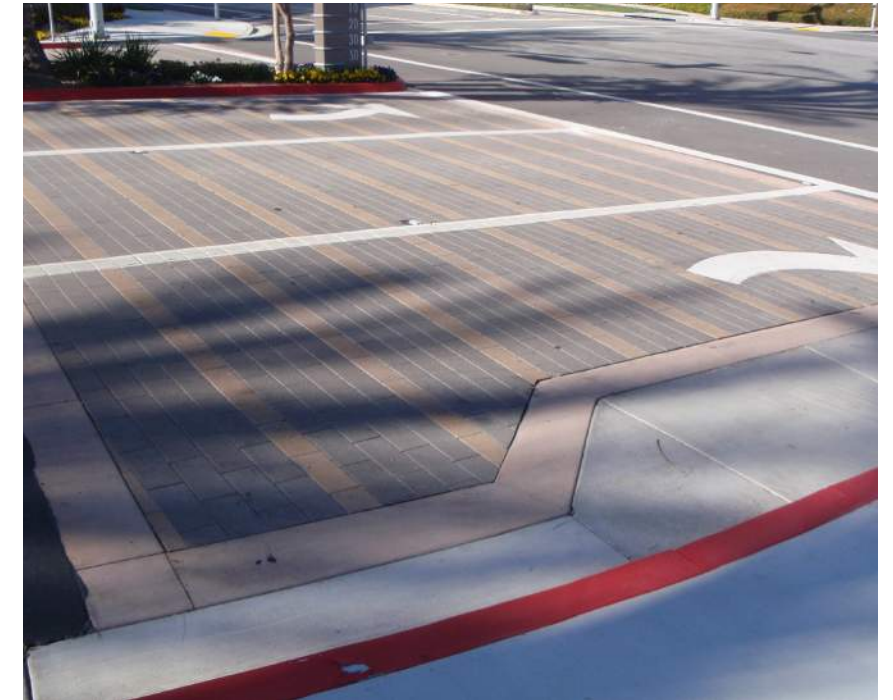
Special paving patterns at pedestrian crossings can increase safety and aesthetic quality.
